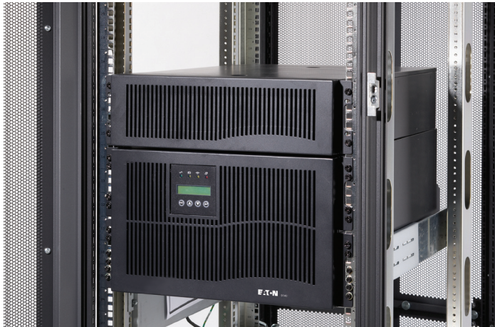
The 9140 and one EBM occupy only 9U of rack space.
